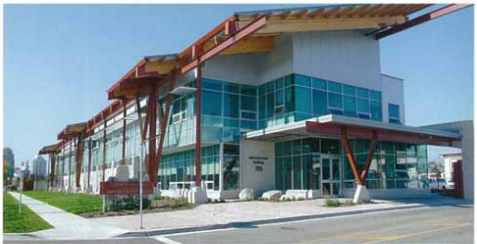
Omicron provided integrated design and construction services for the new $23-million City of Vancouver National Works Yard facility. The Architect of Record was Scott M. Kemp, MAIBC.
