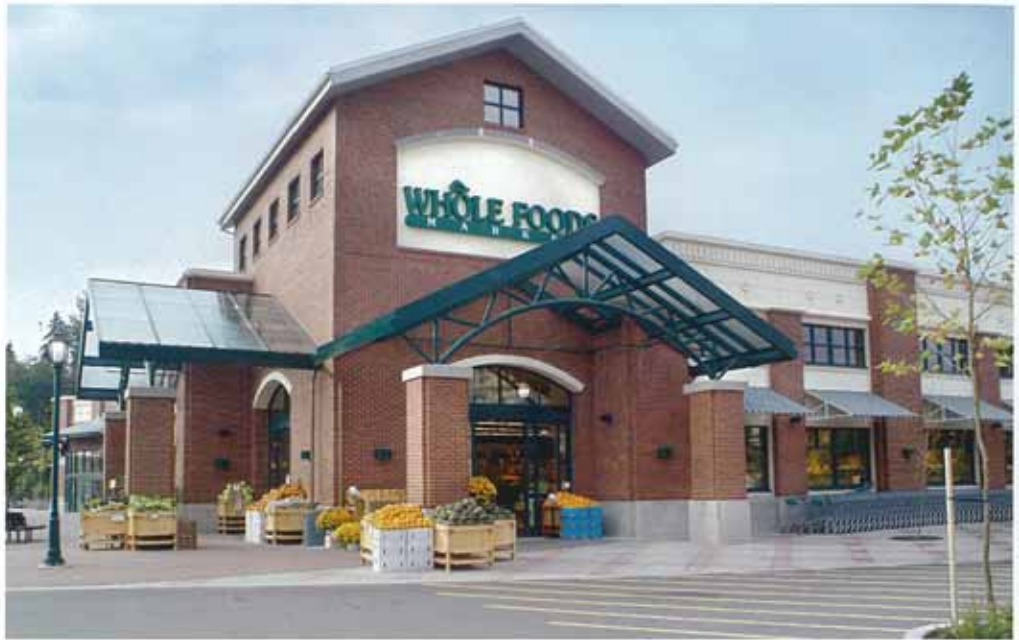
Engineering and construction services for the interior fitout of Whole Foods Market in West Vancouver were provided by Omicron. The Architect of Record was Musson Cattell Mackey Partnership.
